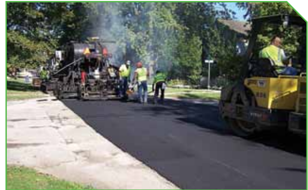
The recycled material levels the previously deformed surface in preparation for an overlay or seal coat.
