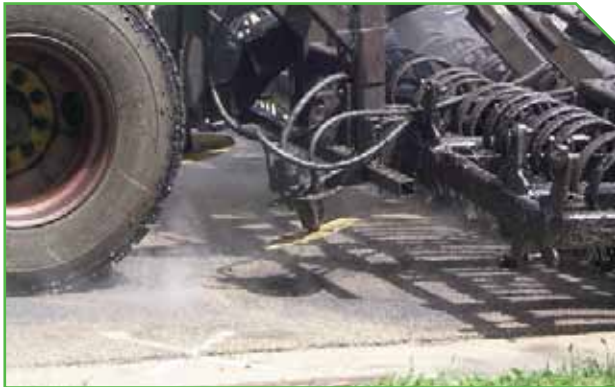
Application of rejuvenating agent improves the viscosity of the aged asphalt.
